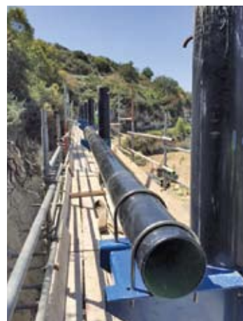
LCR Replacement of pipelines © ISP
