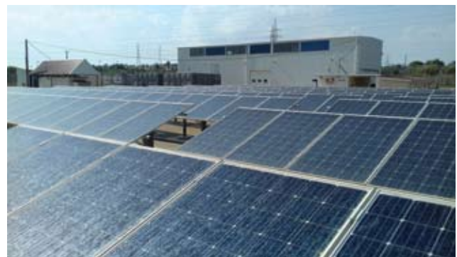
Dhekelia Reverse Osmosis Plant and Photovoltaic Park © ISP
