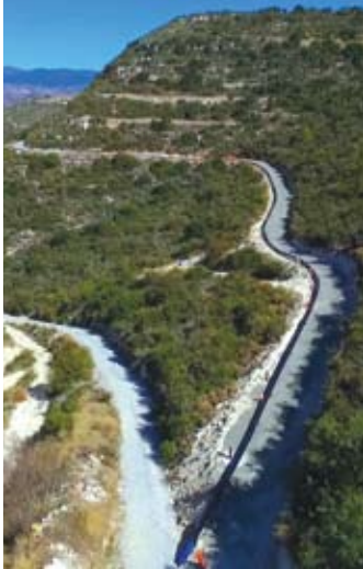
The 532m HDPE pipeline prior to insertion in the tunnel @ISP
