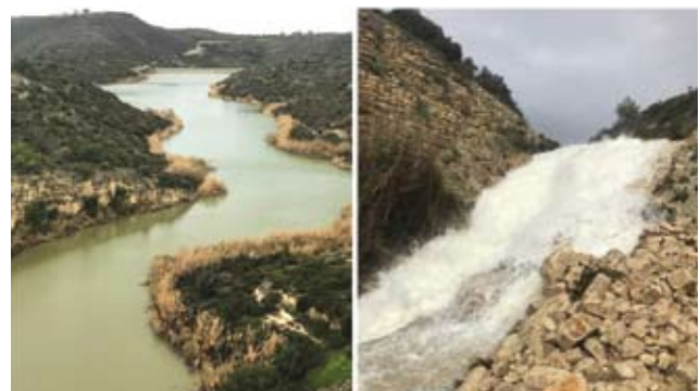
Symvoulos Reservoir and Overflow © ISP
