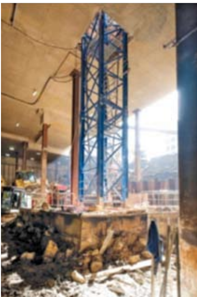
Figure 3 Crane base to be incorporated into the raft of a 3-level basement, built top-down. The initial, localised section of permanent raft (built inside a coffer dam) can be seen
